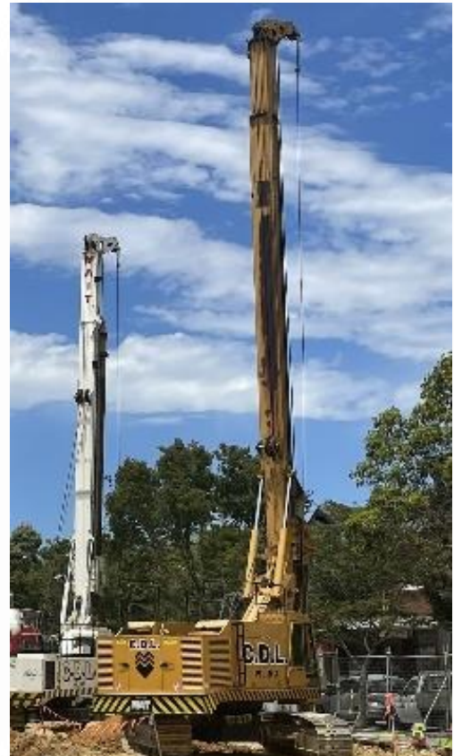
Above: An example of piling rigs used in construction.
