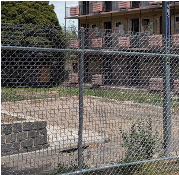
Retaining wall structure
