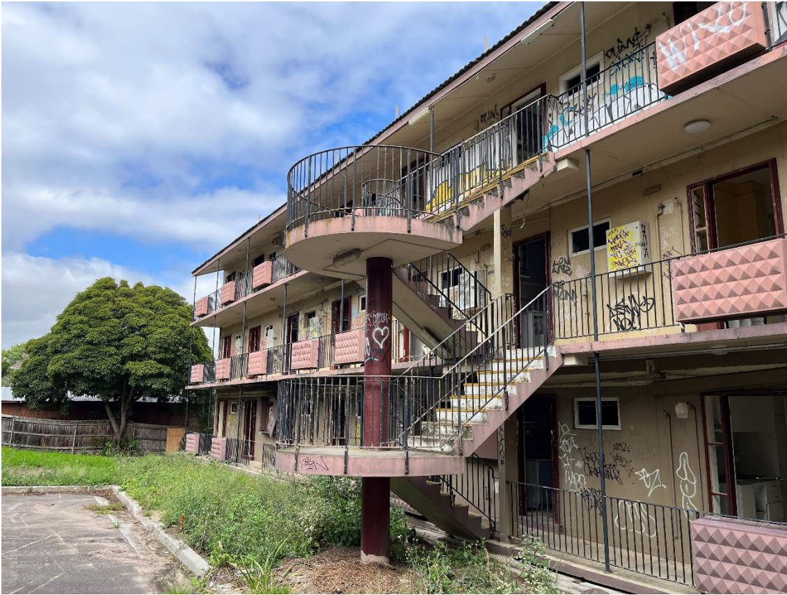
Figure 6 East elevation of 15 Eric Street, access stair to upper walkways
