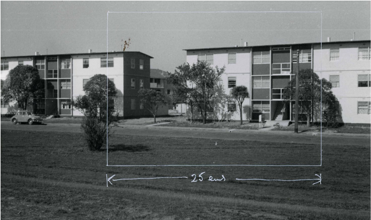
Figure 15 Concrete flats at the Pigdon Estate, North Carlton, view south from Park Street, c. 1957 Source: VPRS 8935, P0001, Unit 3, Public Record Office Victoria
