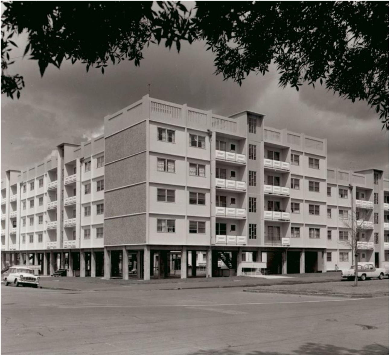
Figure 12 The first group of four-storey walk-ups on stilts with roof-top laundries at Canning Street Carlton Source: State Library of Victoria, Record ID, 9917918593607636 (Wolfgang Sievers photographer, 1962, 'Housing Commission Flats')
