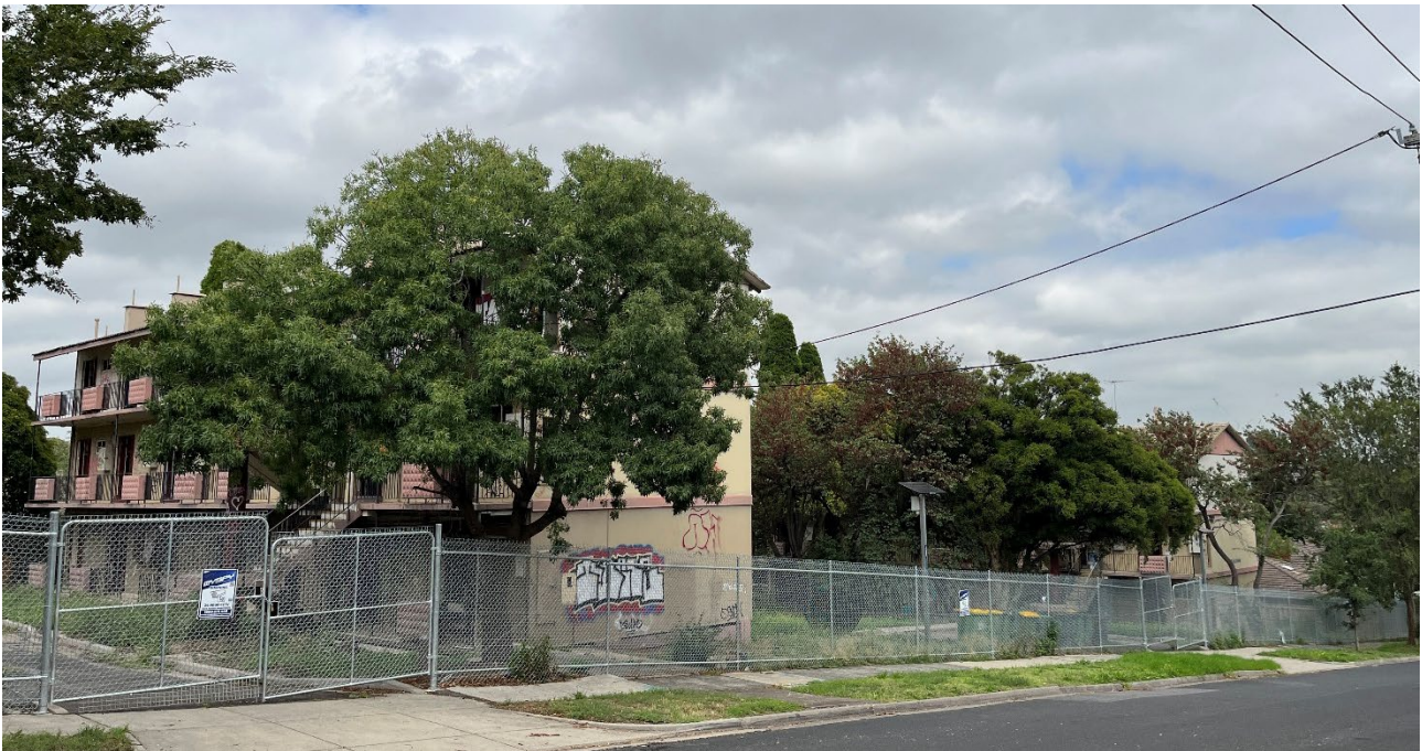
Figure 3 View of the two blocks of flats at the subject site
