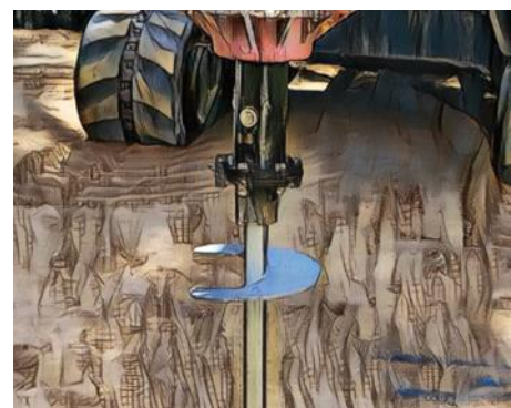
Low impact footings: i.e. - screw piles
